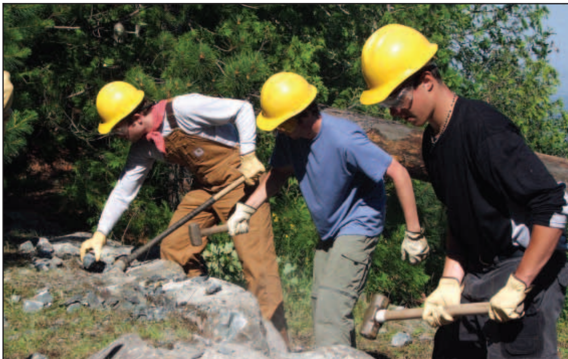
Below: Three crew members use sledgehammers to break apart rocks in order to create gravel to help rebuild the portage trail they are working on.
