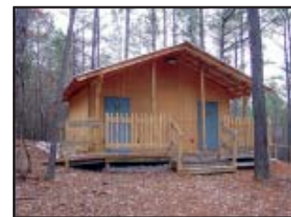
Completed bathroom constructed by the members of Alibamu Lodge, Tukabatchee Area Council
